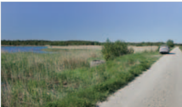
Photo 5.2.3.1. The water exchange of Vööla coastal lake with the sea is prevented by a road built on the coast. The water management plan of the area has assessed the ecological condition of the lake as bad.
