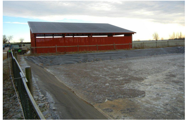
Manure and urine from eating area are scraped to a lagoon and is mixed to a slurry.
