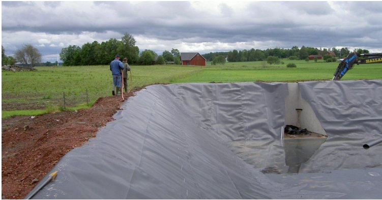
Construction of a lagoon with a liner of non permeable polyethylene.
